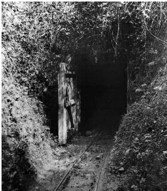
This was the last mine to be worked in Surrey, closed in about 1960 / 61. This was the only entrance, as photographed possibly in the 1930s, but it looked much the same when the author saw it in or about 1959. A single narrow-gauge line of rails ran straight into the hillside for about 400 feet, giving access via turntables to several headings, where stone was extracted, at right angles on the left-hand (west) side. A plan of the then active mine was made in 1941 by the Reigate borough engineer, presumably for possible use as an air-raid shelter. It shows that the tunnelling then in use has been driven through previously mined ground nearer the entrance and on the east side, indicated sketchily as 'old workings'.
